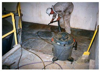
At this chemical storage area in a large Boston hotel's laundry, chemical corrosion had severely damaged the diamond plate platforms.
