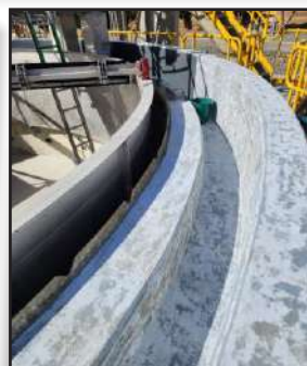
2. DuraQuartz used on the surface.
