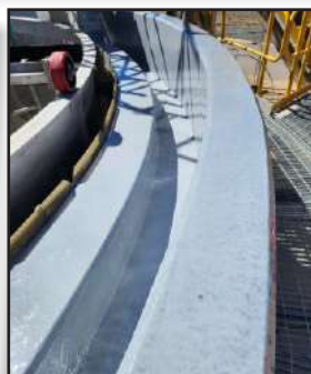
3. First coat of CHEMCLAD GP.
