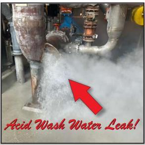
This paper mill in North Carolina was being restarted after a two-week maintenance shutdown. One critical process pump moving acid wash water was being put back into service, and the water pressure and flow volume created a "water hammer" against the inner walls of the pipe's elbow section. This caused the elbow to become the "fail point" of the pipe, resulting in a massive leak.
