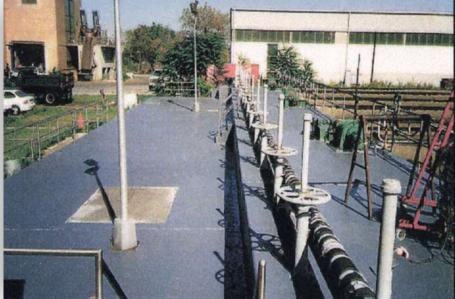
system. Under the watchful eyes of ENECON North East's Field Engineering Team, all cracks in the concrete decks were first repaired with ENECRETE DuraQuartz and then the entire area was protected with CHEMCLAD GP.
