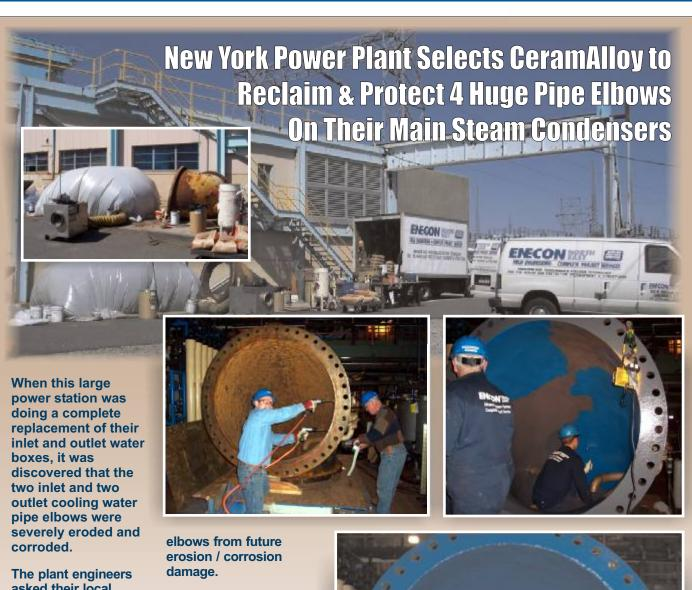
asked their local **ENECON North East Engineering Team to** remove the heavy scale and graphitization and then repair all the pitted areas with CeramAllov CP+AC. Two coats of CeramAlloy CL+AC were then applied to completely resurface and protect these 54 inch diameter
